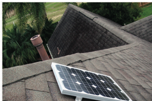
Standard Mounting Bracket installed on shingled roof
